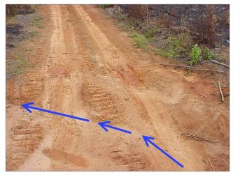
The diverted water is carried off the road and through the wing ditch into a vegetated patch of land which will absorb the runoff.
